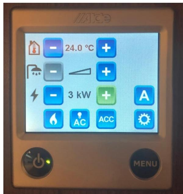
Choose the desired temperatur and effect and the gas off. Press the gear at the bottom right corner.
